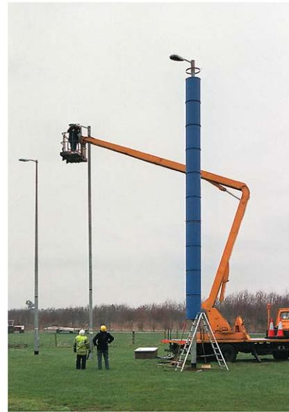
Fig. 5. Plastic drums used to enlarge the diameter of one of the lighting columns.
