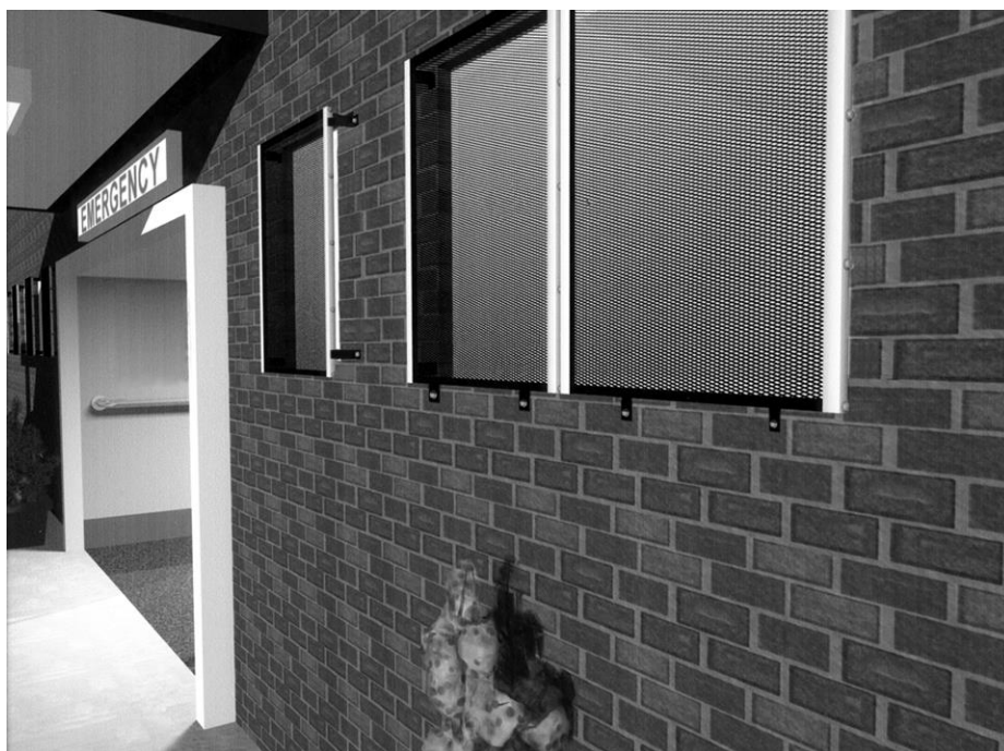
Figure 1. Installation of a Stormgard missile protection screen
